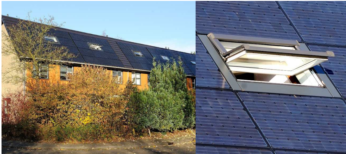
FIGURE 22. STAFIER STANDAARD AS AN IN-ROOF MOUNTING SYSTEM (MAARN, THE NETHERLANDS), 29 TERRACED DWELLINGS
