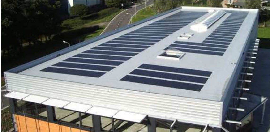
FIGURE 10. PV MEMBRANES EMBEDDED IN A FLAT ROOF COVER (SOURCE: WEKA DAKSYSTEMEN).
