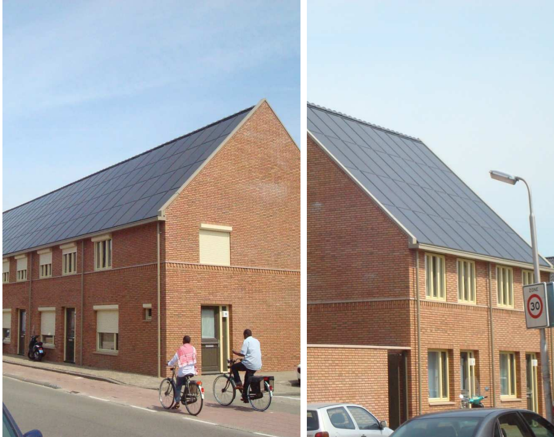
FIGURE 23. SCX SOLOROOF AS BIPV FULL ROOF SOLUTION (TILBURG, THE NETHERLANDS), 75 TERRACED DWELLINGS
