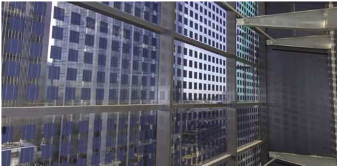
FIGURE 12. THE "HERON TOWER" IN LONDON WITH THE SEMI-TRANSPARENT DOBLE SKIN -BIPV FAÇADE (PICTURE: P. BONOMO).
