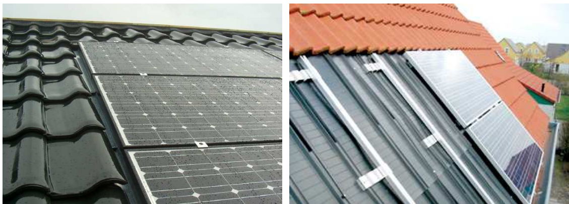
FIGURE 5. EXAMPLES OF IN-ROOF MOUNTING SYSTEMS ARE USED IN SLOPED ROOFS (SOURCE: RENUSOL INTERSOLE)
